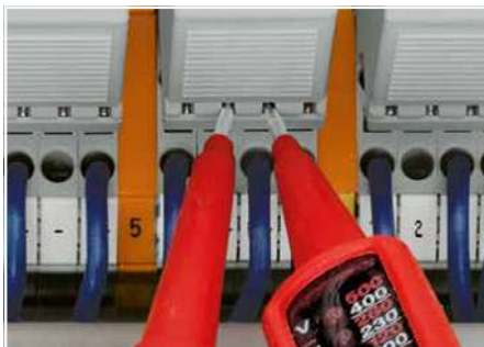
Function testing via touch-proof test slots.
