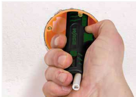
Stripping a cable sheath.
