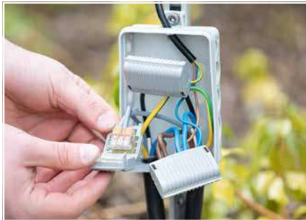
Connecting a bollard light
