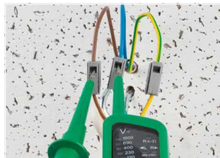
Testing via separate test ports.
