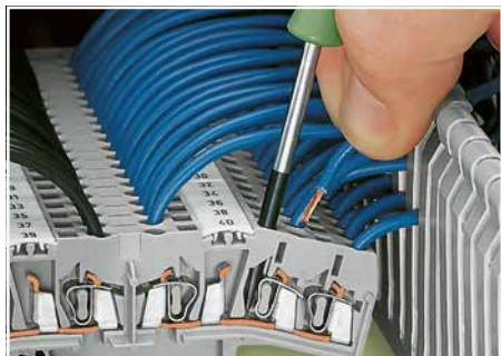
Terminal blocks for matrix patching: Inserting/removing a conductor on the terminal block's side-entry. With ferruled conductors, it is necessary to use a terminal block one size smaller than the conductor's nominal cross section.
