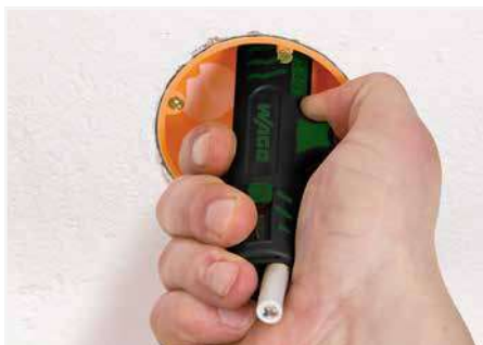
Stripping a cable sheath.
