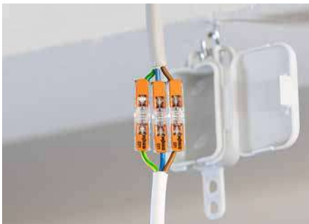
Lighting connection in suspended ceilings
