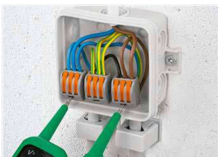
Testing the wired connectors.
