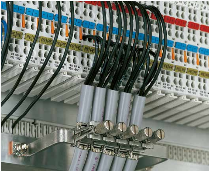
U-shaped (10 x 3) mm copper busbar
