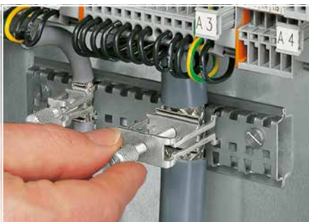
Tightening/removing a shield clamping saddle.
