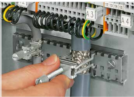
Securing an additional shield clamping saddle.
