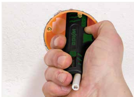
Stripping a cable sheath.
